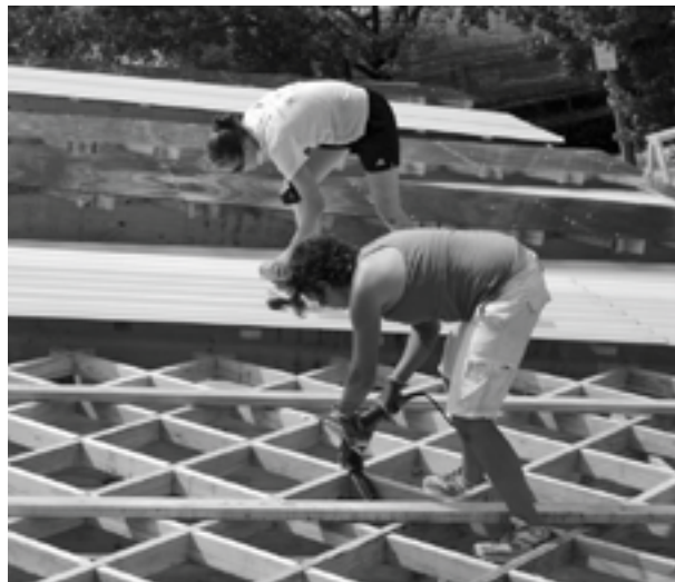
Mass Art students do roofing on the Carter School bus shelter.
