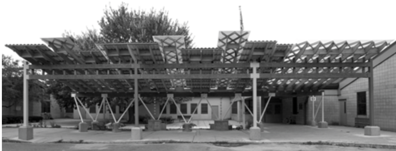
The finished project: After a downpour (note the puddles in the foreground), the interactive rain garden is deemed a success.
